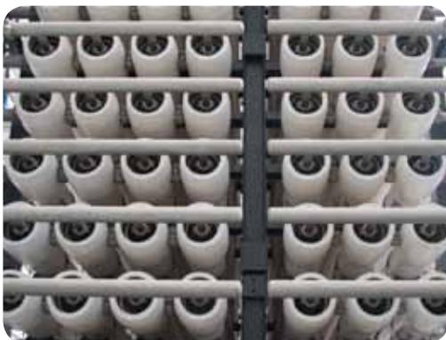
With a total production of 22.900 m<sup>3</sup>/day, the plant consists of three skids with 2 stages and a total recovery of 55%. The facilities were built with enough space to double the production in future expansion if it is needed.
